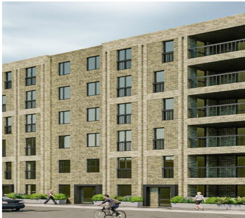
(Sansom Road – CGI of completed scheme)
